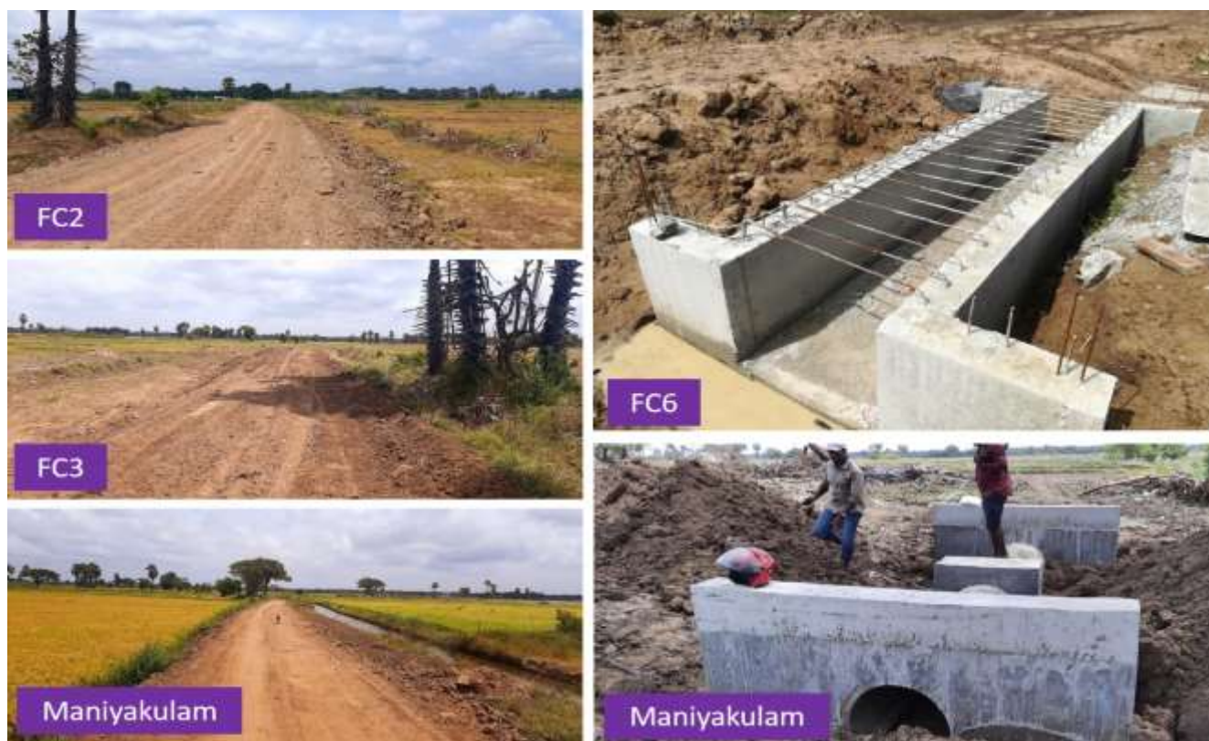
Fig.20: Current status of Vanneri Agri- road construction
