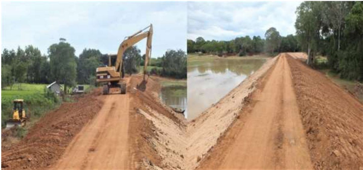
The rehabilitation works on the Ranawaranawa tank and canal system
