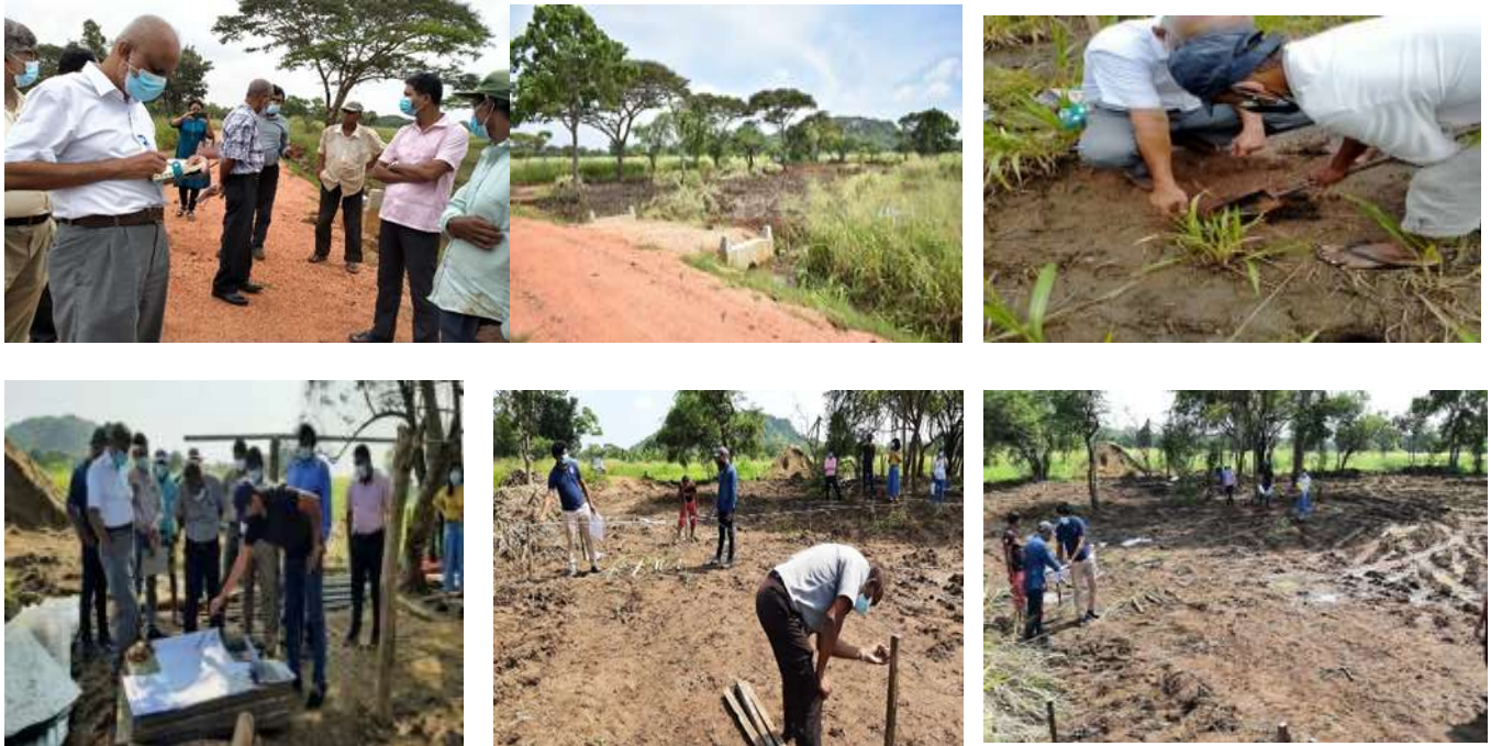
Visit WB Country Director to Thirappane FFS & laying the foundation
